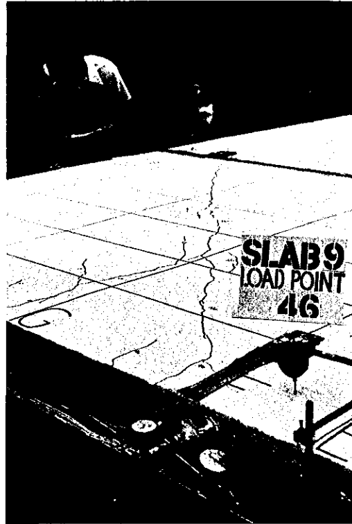
(b) DIAGONAL CRACK AT NE CORNER (LP 46).
